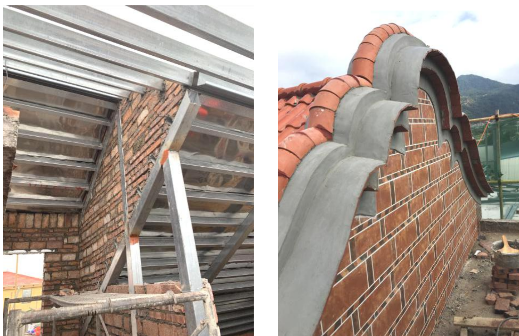
(a) 钢梁上砖砌围护墙
